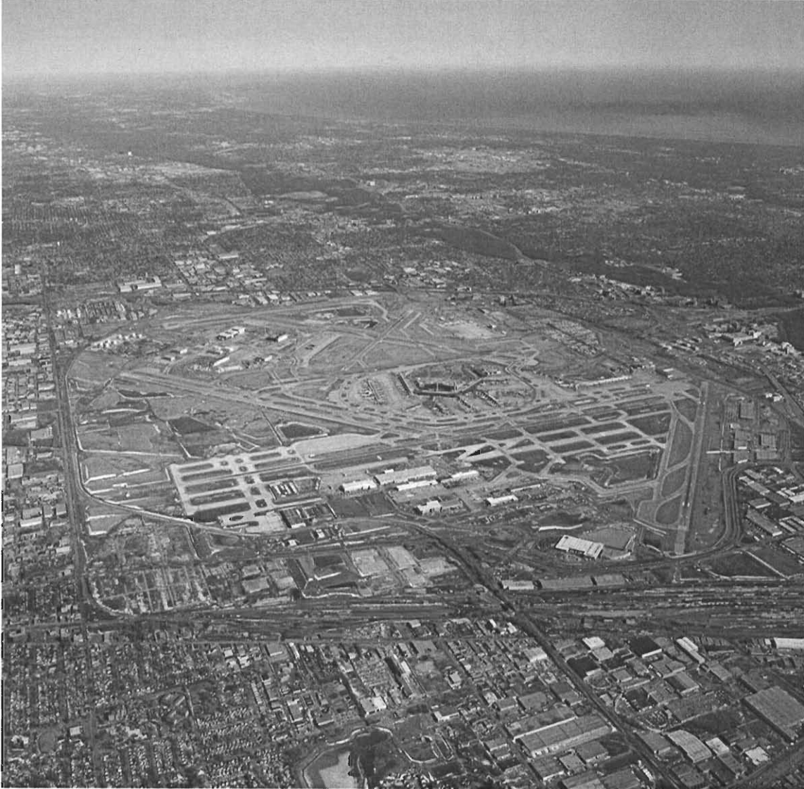
Figure 3.2 Aerial Photograph of O'Hare International Airport Photo Source: Seita, 2012. http://www.flickr.com/photos/jseita/5457379097/
